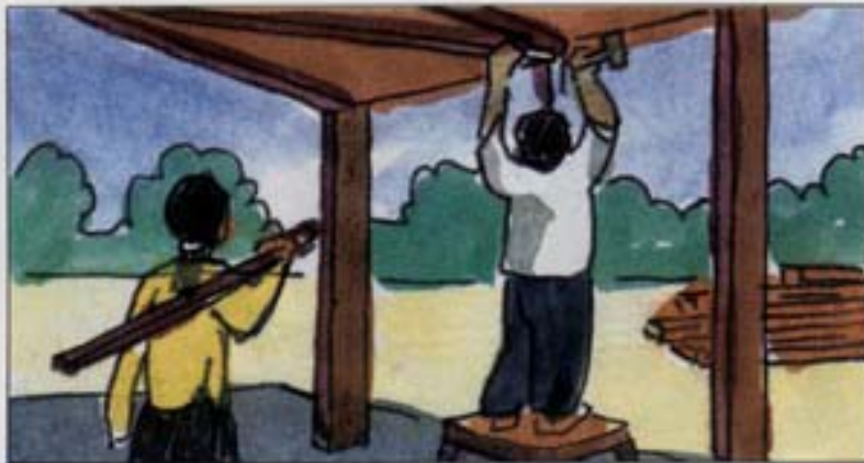
The inside of the veranda has diagonal bracing put in to stop the wind twisting it out of shape.
